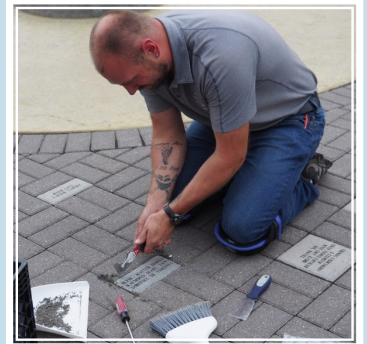
Above: Anthony Helmer from McGough installs the pavers
